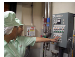
Members of Komaki Plant's energy conservation project examining facilities on-site
