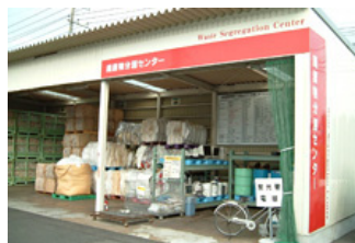
Nasu Plant's recycling center
