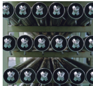
Reverse osmosis (RO) condensation system
