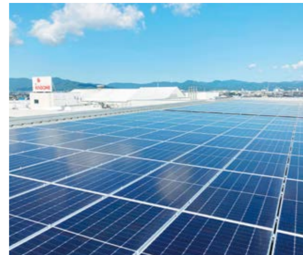
Solar panels at the Kozakai Plant
