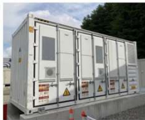
Storage battery system installed at the Fujimi Plant
