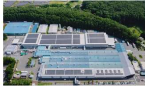
Fujimi Plant's rooftop solar power generation system
