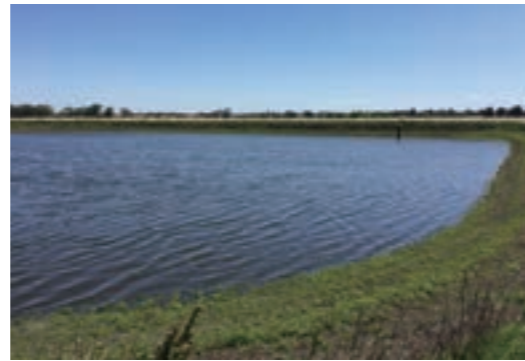
Reservoir dam of Kagome Australia Pty Ltd.
