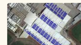
Installation of solar panels
