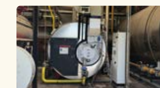
Installation of new-type boiler
