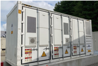
Storage battery system at the Fujimi Plant
